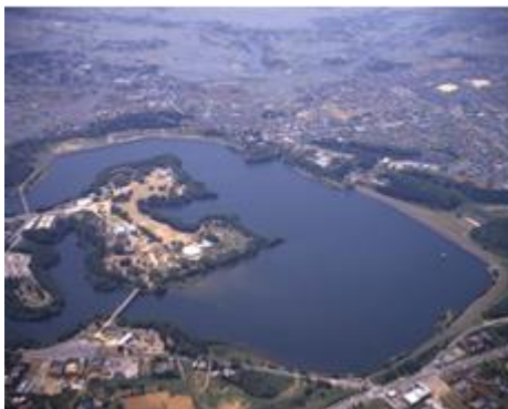
Aerial view of the Yamakura Dam site
